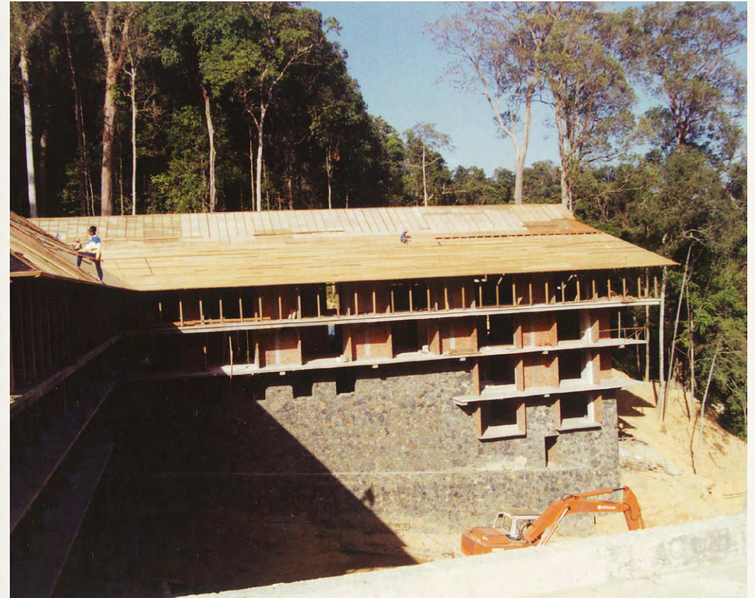
Construction of the Main Building, 1992.
