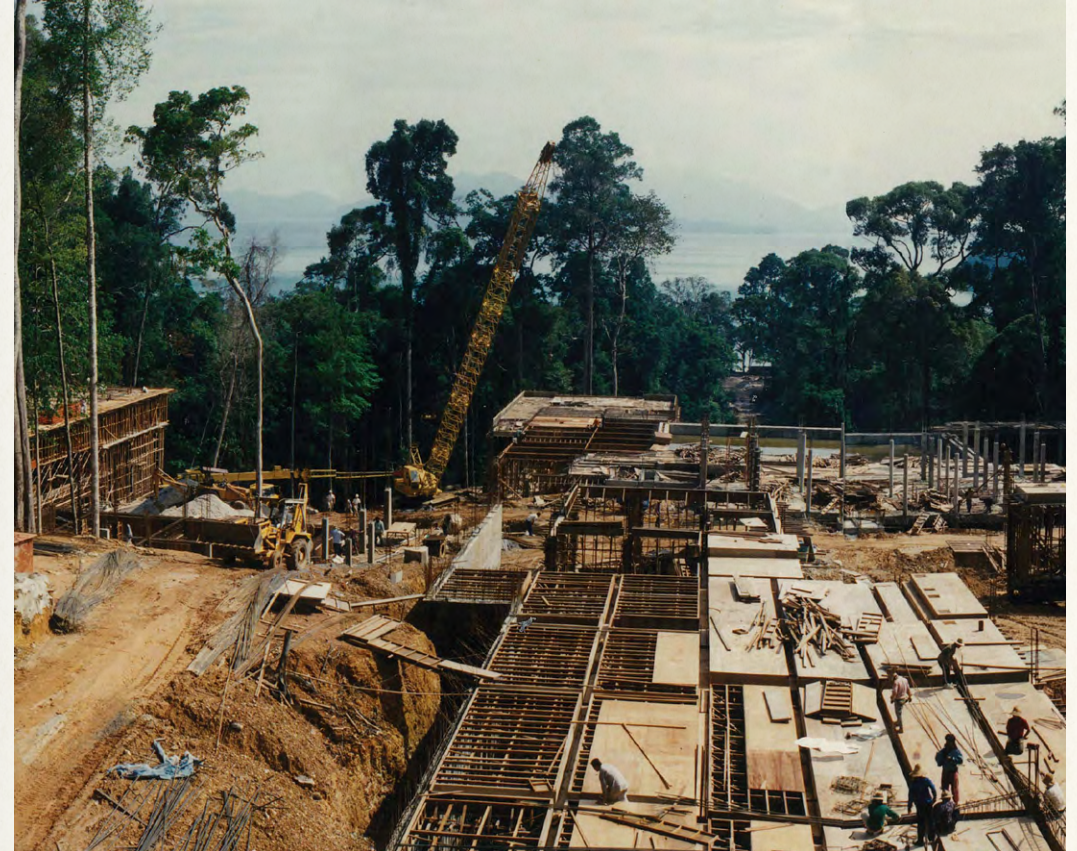
Construction of the Main Building, 1991.
